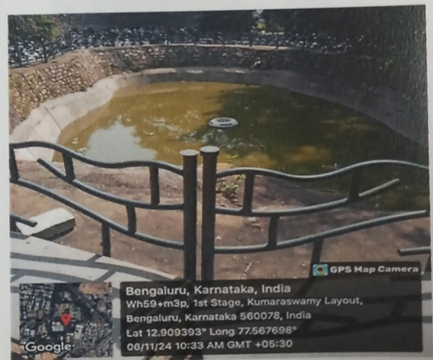
COLLECTED WATER BEING DRAINED AND DISTRIBUTED
